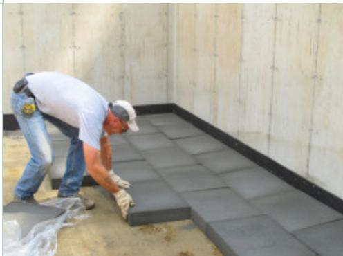
Avoidance of flame retardants was one of the primary reasons the author used Foamglas (4" layer) under the slab in his new house. Its high compressive strength makes this a good option, though it is more than twice the cost of XPS.
